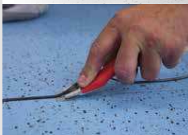
GTI EL5 CLEANTECH - WELDING CONDUCTIVE ROD
